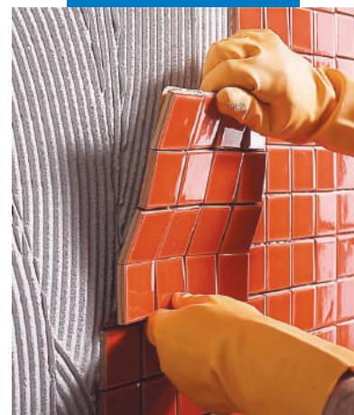
Installation of mosaic ceramic on wall
