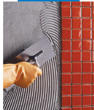
Installation of mosaic ceramic on wall
