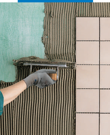
Laying on gypsum treated with Primer G
