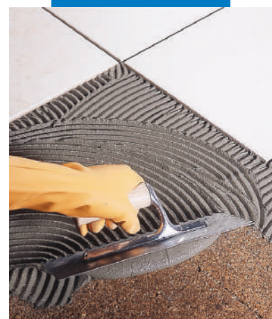
Installation of single-fired tiles on cork
