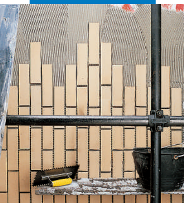
Exterior wall fixing
