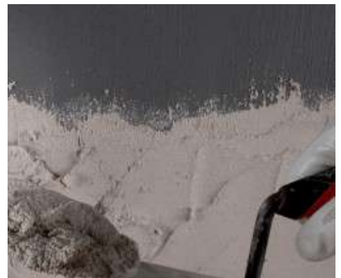
Application of render on Eco Prim Grip Plus
