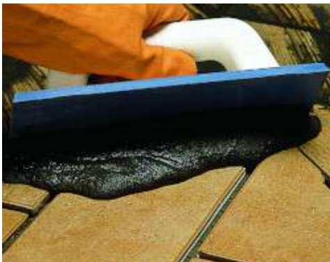
Grouting an external klinker tile floor with Keracolor GG mixed with Fugolastic
