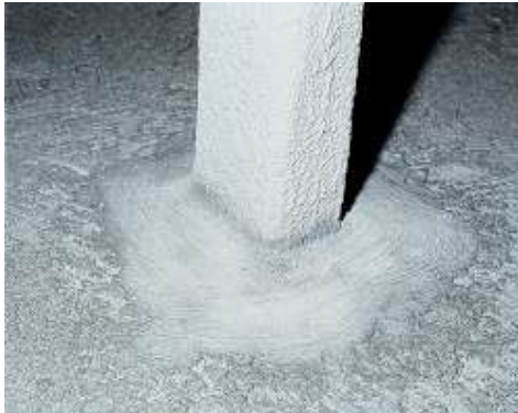
Pillar waterproofed with Idrosilex
