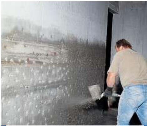
Spraying on the first coat of mortar admixed with Idrosilex Liquid
