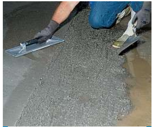
Screeding with mortar admixed with Idrosilex Liquid
