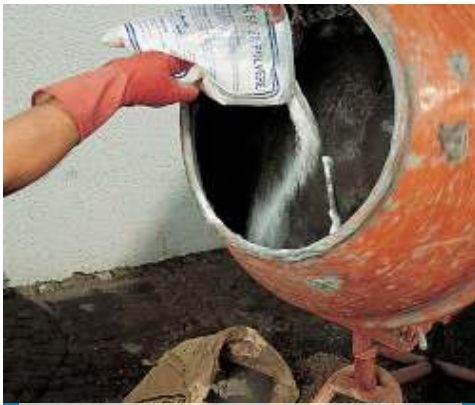
Preparing waterproof mortar admixed with Idrosilex Powder
