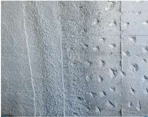
Applying mortar admixed with Idrosilex over concrete roughened with a bush hammer
