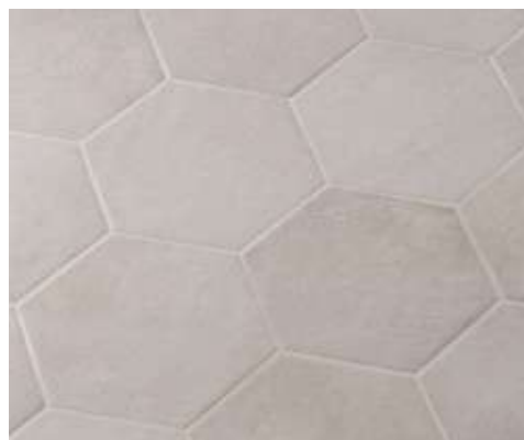
Floor grouted with Keracolor FF
