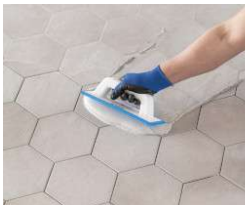
Application of Keracolor FF with MAPEI float
