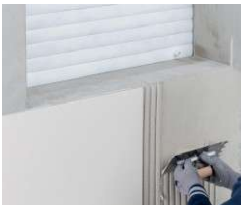
Installation of large-size ceramic tiles
