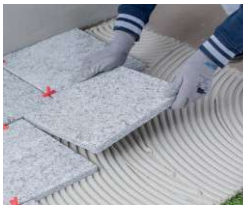
Installation of natural stone in exterior
