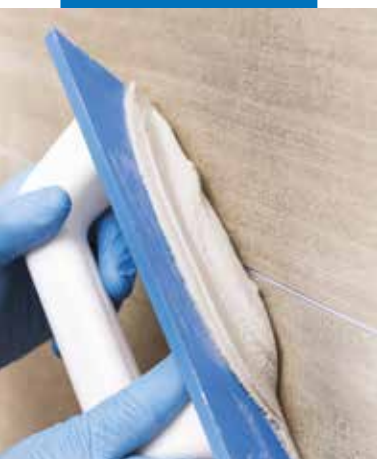
Applying Kerapoxy 4 LVT with a rubber trowel
