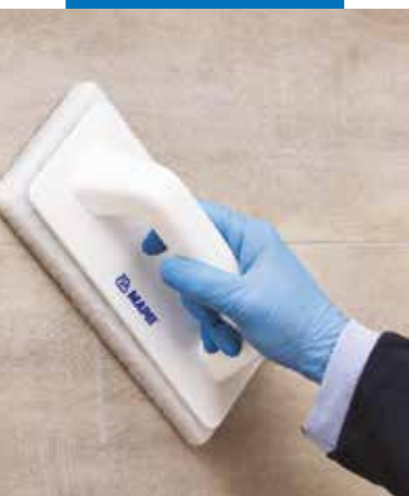
Initial cleaning with Scotch-Brite®
