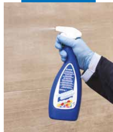
Cleaning where required with Kerapoxy Cleaner
