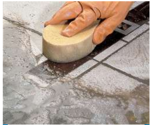
Finishing a ceramic tile floor with wood inlays with a sponge
