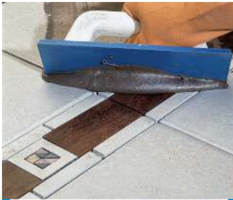
Grouting a ceramic tile floor with wood inlays with a trowel
