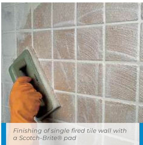
Finishing of single fired tile wall with a sponge
