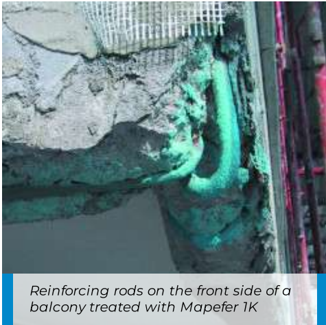
Demolition of degraded concrete
