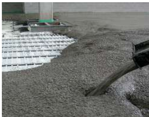
Pouring concrete with the addition of Mapefibre NS18 to counter plastic shrinkage
