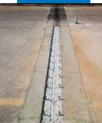
Repairing a joint of a highway bridge with Mapefill
