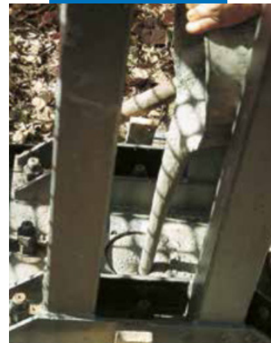
Anchoring with mortar Mapefill
