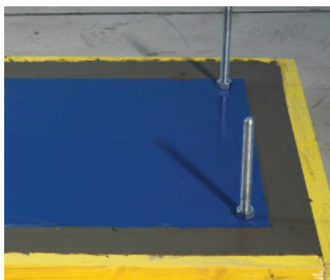
Completed grouting of anchor bolts with Mapefill R
