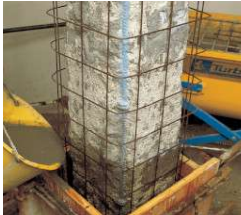
Pouring into a formwork
