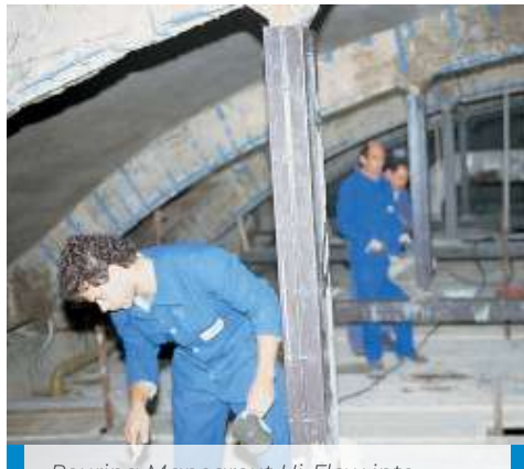
Pouring Mapegrout Hi-Flow into metal formwork
