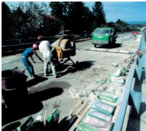
Reforming road joints
