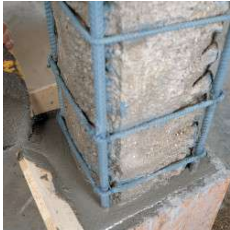
Removing wooden formwork
