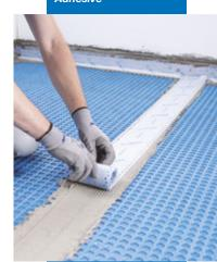
Waterproofing of joints between the sheets with Mapeband Easy, bonded with Mapeguard WP Adhesive
