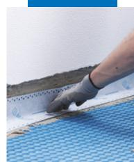
Perimetral waterproofing with Mapeband Easy, bonded with Mapeguard WP Adhesive
