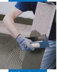
Install ceramic or stone tiles with a suitable MAPEI adhesive of at least C2 class
