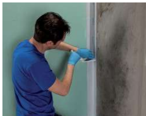
Application of Mapeband PE 120 using Mapegum WPS
