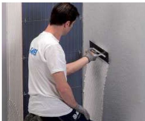
Installing wall covering using Keraflex Maxi S1
