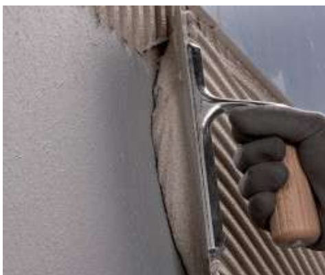
Installing floor covering using Ultramastic III
