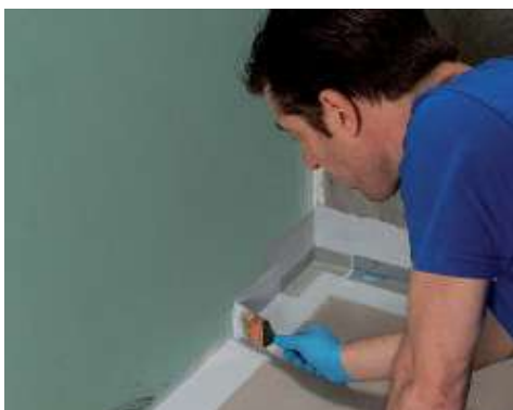
Application of Mapeband PE 120 using Mapegum WPS
