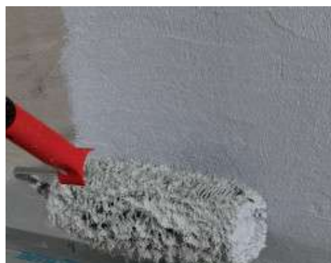
Application of Mapegum WPS with a roller
