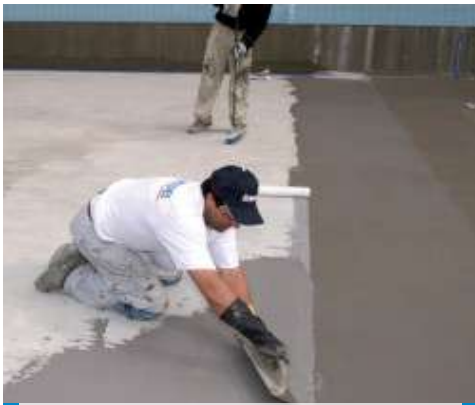
Waterproofing a swimming pool with Mapelastic
