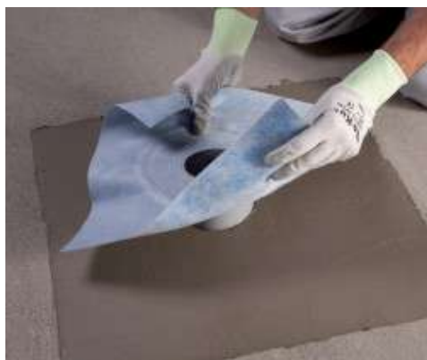
Application of Drain Vertical on Mapelastic
