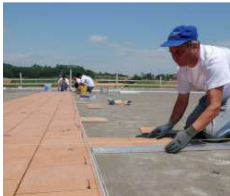
Installing ceramic with Kerabond + Isolastic
