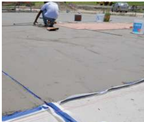
Waterproofing screeds with Mapelastic and Mapeband
