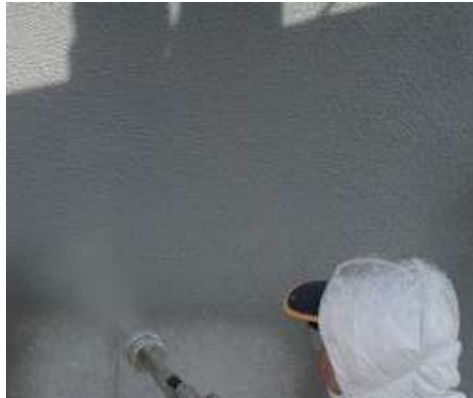
Example of Mapelastic applied on a viaduct by spraying
