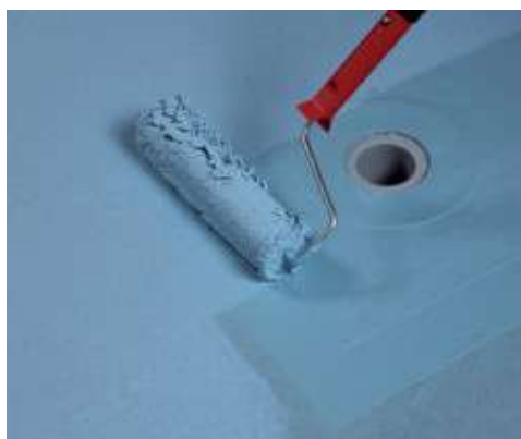
Application by roller of the second coat of Mapelastic AquaDefense
