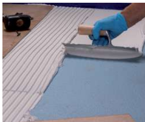
Bonding tiles on Mapelastic AquaDefense
