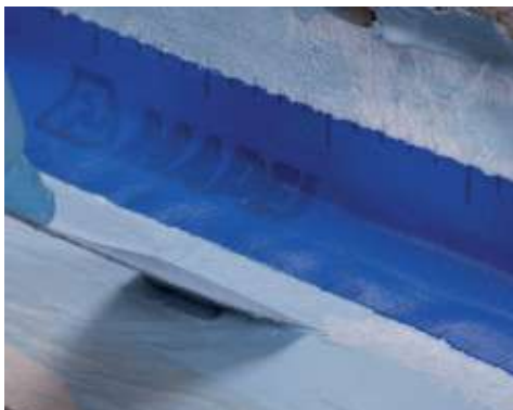
Application of Mapeband on a wall-floor fillet joint with Mapelastic AquaDefense
