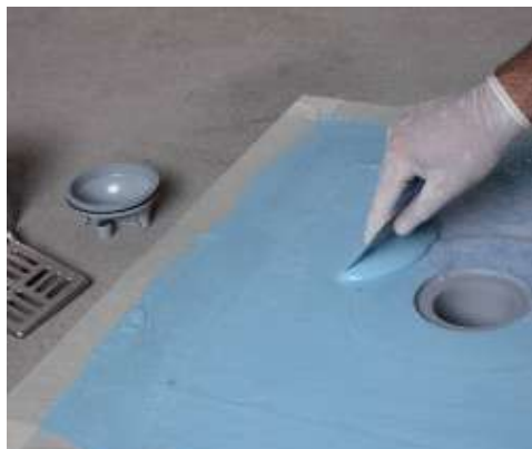
Impregnating Drain Vertical fabric with Mapelastic AquaDefense
