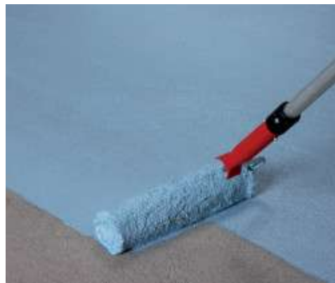
Application of the first coat of Mapelastic AquaDefense on a screed
