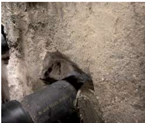
Confining Mapeproof Swell with Mapegrout T40
