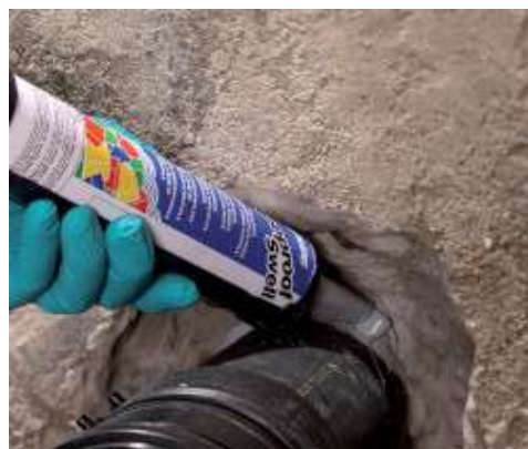
Applying Mapeproof Swell around a pipe
