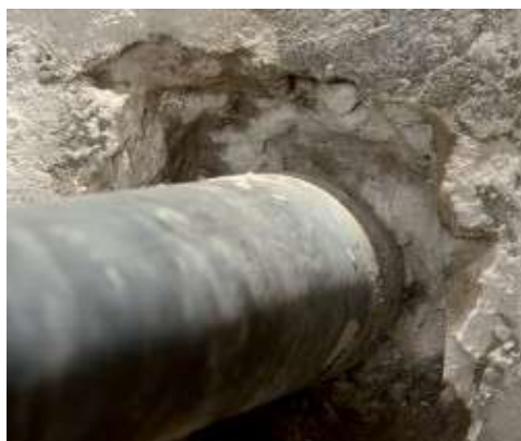
Breaking out the structure around a pipe
